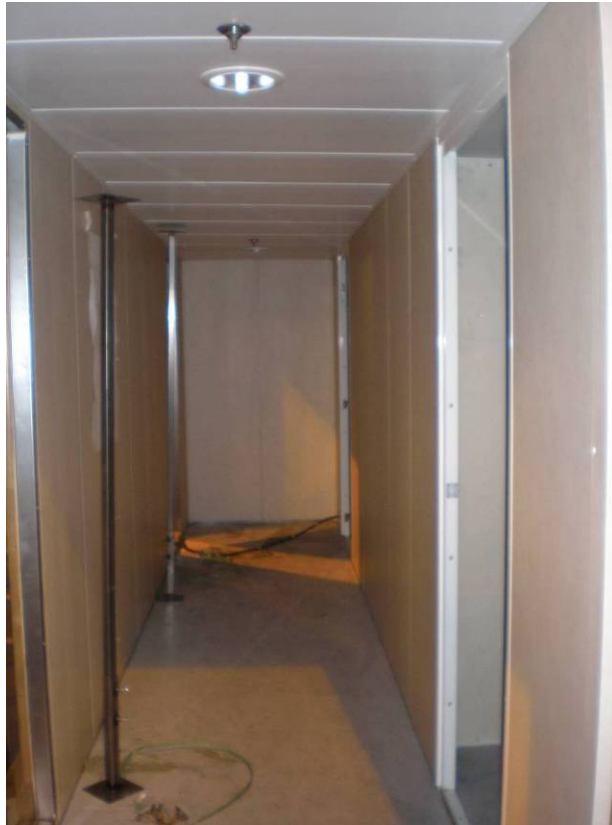
Figure 4-13 Photo showing the corridor and entrances to the two cabins
